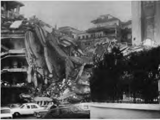
Apartment Damaged by Israeli Bombardment (Feb., 1983).
